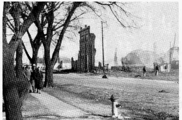
The west wall of the liquor store remains standing, a lonely reminder of what used to be.
