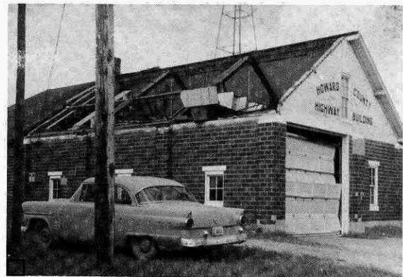
Howard County Highway Building
