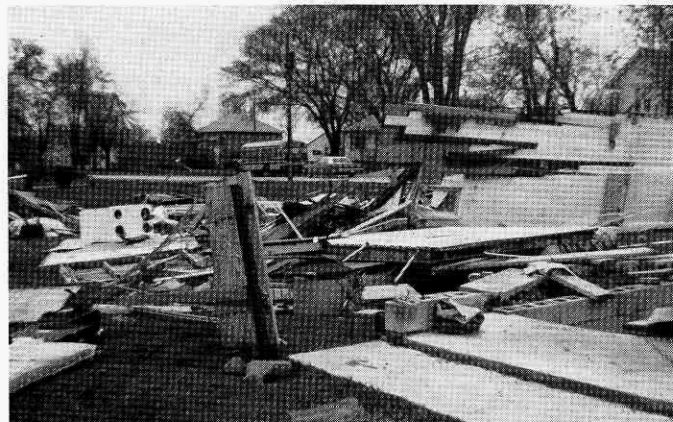
The remains of the Tom Smith home in the northwest part of town.
