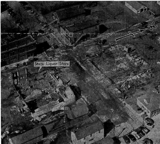
Don Ultang, Des Moines Register-Tribune pilot-photographer, snapped this photograph over Elma late Thursday morning after firemen had brought the destructive blaze under control. The fire burned out a two-block area on both sides of Elma's main street. Visible in this photograph are Klobassa's grocery, the Peoples' State Bank, the Elma Cooperative Creamery and the Hopkins Hatchery, creating a boundary of undamaged buildings surrounding the devastated area.
