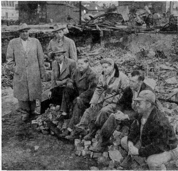
Visiting the scene of their losses are seven men who lost property and businesses when a $250,000 fire destroyed a considerable area of the west side business district in Elma March 4. From left are E. B. Richmond, Charles Jones, Leo Tonn, Bob Jacoby, C. G. Stratton, Dan Conway and Reuben Tuchek. There is little hope the buildings will be replaced.
