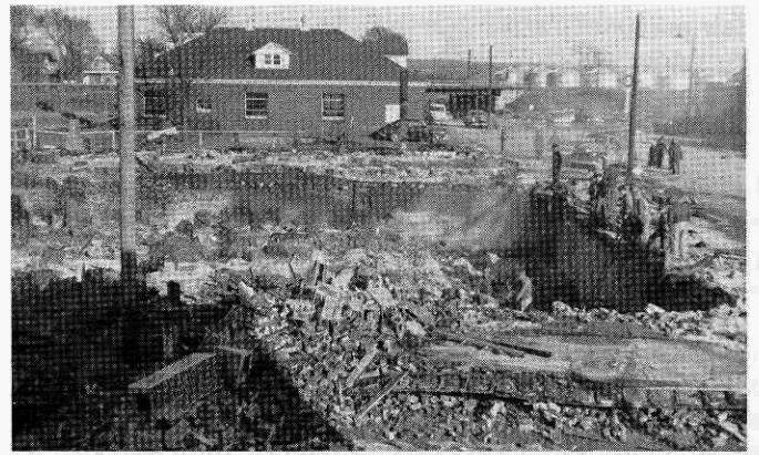
This large hole is all that remains of the five businesses that were located on the north side of Main Street. The Elma Co-operative Creamery is in the background.
