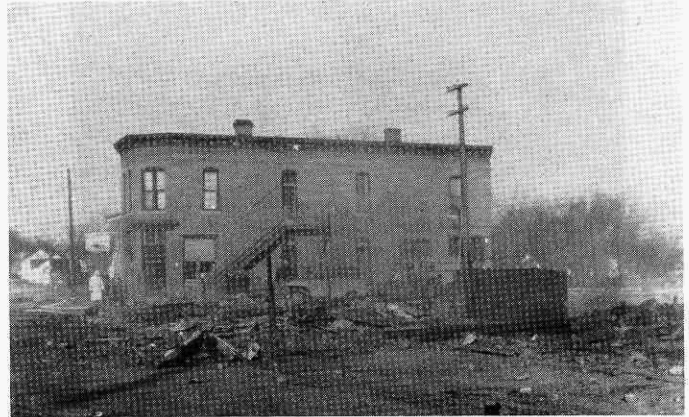
People's Savings Bank can be seen in the background, while in the foreground is the rubble left from West Side Tavern and Tonn's Clothing Store.
